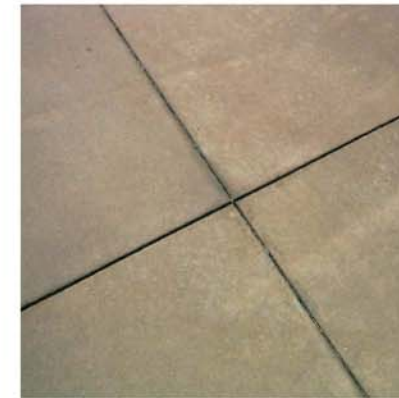
Integral Colored Concrete
